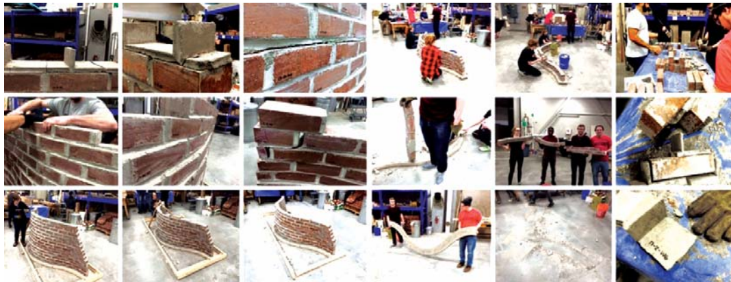
Figure 3. Four weeks of collaborative wall deconstruction and material cataloguing of the first ruled surface brick wall built in the spring of 2016.
