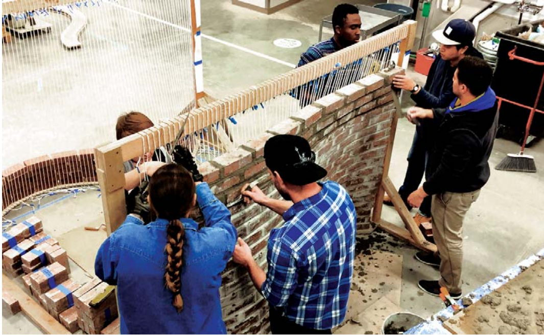
Figure 1. Students working on version two of ruled surface brick wall against string and wood formwork.
