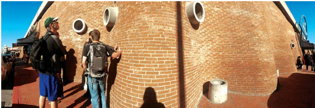
Figure 4. Panorama of ruled surface wall on the North side of the Montevideo Shopping Center in Uruguay.
