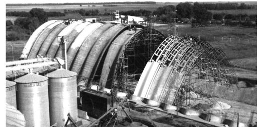
Figure 5. Disengaging the encofrado and preparing to set the tenth vault on the east side of the Silo CADYL. Images by Dakota Mathews-Schmidt and Tyson Vogt.
