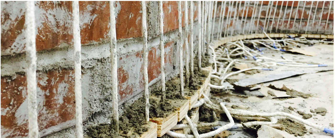
Figure 1: Bottom brick courses of Ruled Surface wall with string guides..
